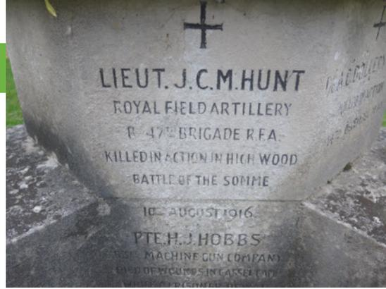
treatment is now required. The stonework has become heavily weather stained exacerbated by the damp location and weather action has also caused the lettering to become seriously eroded. In addition, the base is in need of minor repairs to the stonework with joints re-pointed where mortar has become dislodged.
